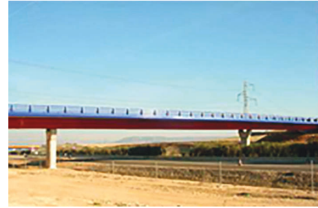
FIGURE 1: The Magaz bridge.
