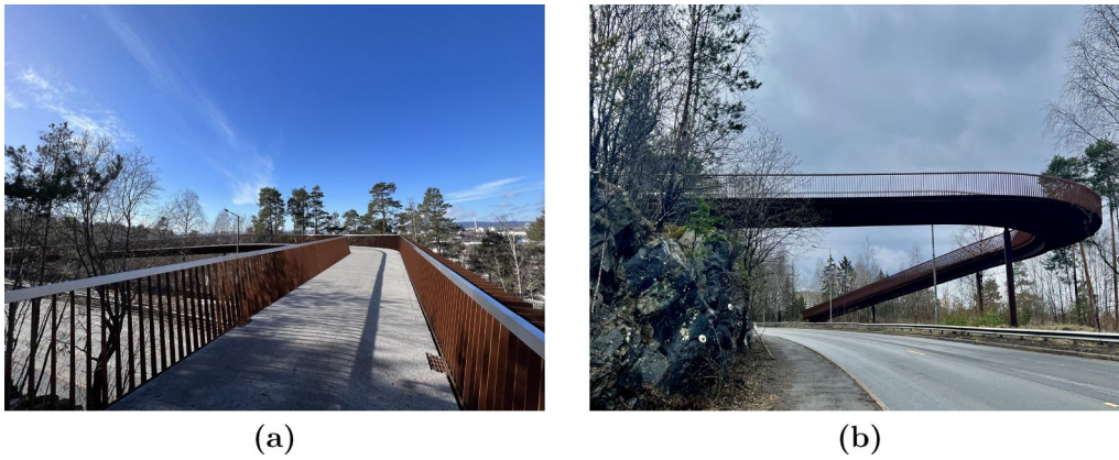
Figure 3. Bumerang footbridge in Oslo, Norway.
