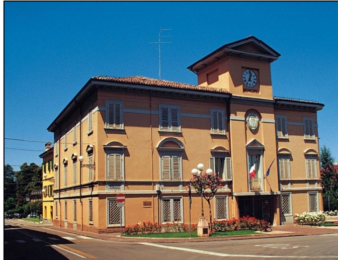
Figure 11-3 Current Fiorano Modenese's Town hall seat
