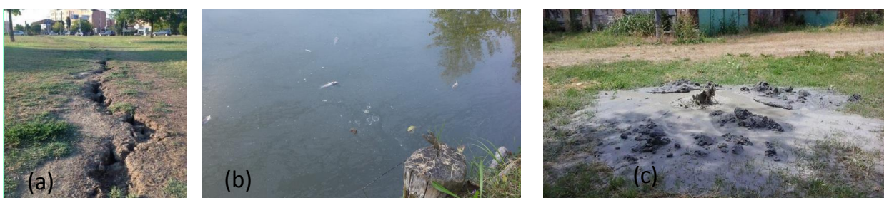
Figure 4.4-4. Picture showing examples of unusual manifestations. (a) The alarm date from August 2013, it is located in the urban area of Ferrara and it shows an important terrain fissure apparently similar to the fissures or cracks induced by the 2012 seismic sequence. (b) The alarm dates from September 2014, it is located in the district of Crevalcore (BO) and it concerns relations to anomalous fish death. (c) The alarm dates on May 2014 and it was located in the district of Bondeno. It shows an example of sand boil. (Photo taken by Giovanni Martinelli). ( http://mappegis.regione.emiliaromagna.it/gstatico/documenti/Segnalaz_Fenomeni_Terremoto/ ).
