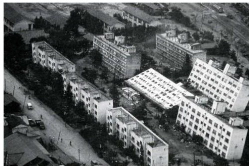
Figure 3.1-9 Example of Damage from liquefaction. Niigata earthquake (1964).
