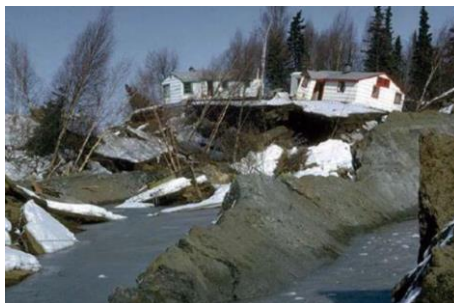
Figure 3.1-6 Example of flow failure of slopes. Flow failures of slopes involving very large down-slope movements of a soil mass. Turnagain (1964) Alaska.
