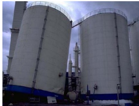
Figure 3.1-8 Example of Damage from liquefaction. Kocaeli (1999) Turchia.
