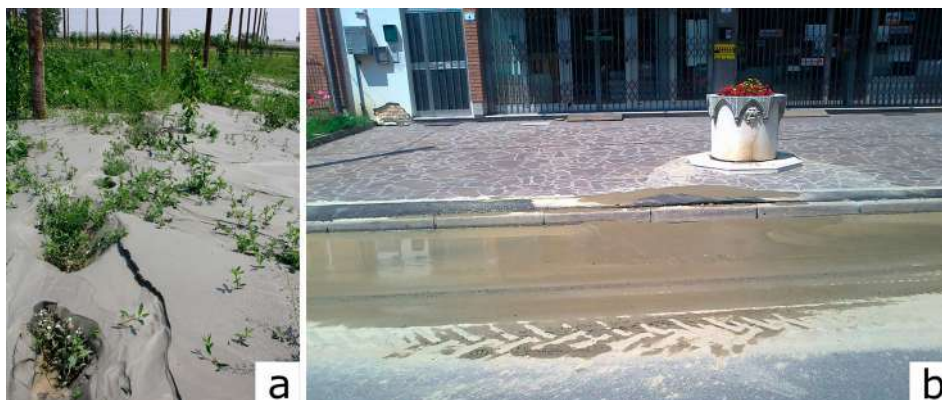
Figure 4. Examples of liquefaction induced by the earthquake of 29th May 2012 in the surroundings of Quistello (a) and in the urban centre of Moglia (b), respectively within the eastern and central sectors of the Main Map .
