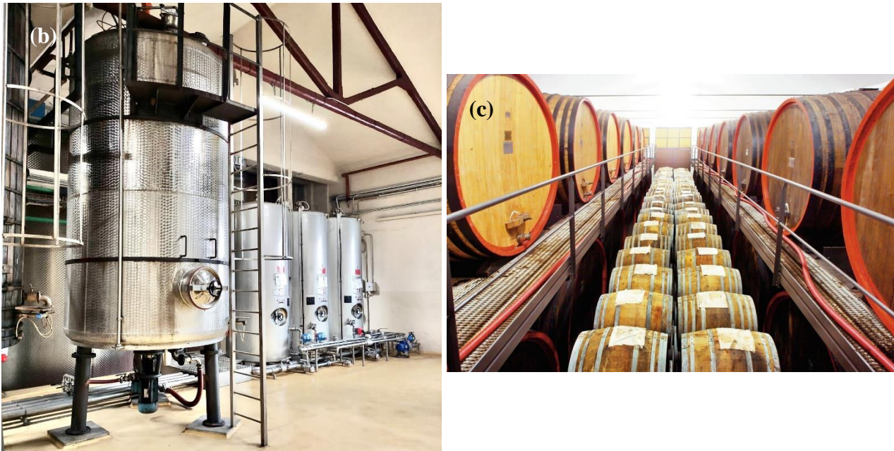
Figure 1.8 (a) Overview of the main plant of Ponti SpA in Ghemme (NO) (b) Frings used for the production of vinegar in Ghemme plant (c) Wood vats presents in Vignola (MO) plant for the production of Balsamic Vinegar of Modena P.G.I.
