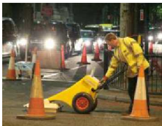
(b) Roadway inspection.
