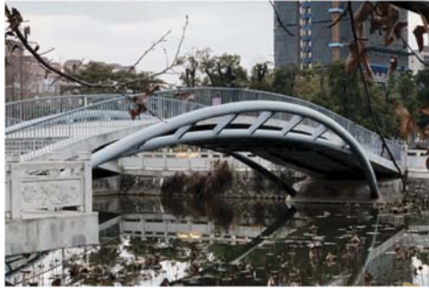
Figure 1. A stress-ribbon CFST arch pedestrian bridge at Fuzhou university.
