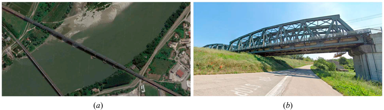
Fig. 1. Ostiglia-Revere viaduct: (a) top view and (b) example span street view from Google Earth.
