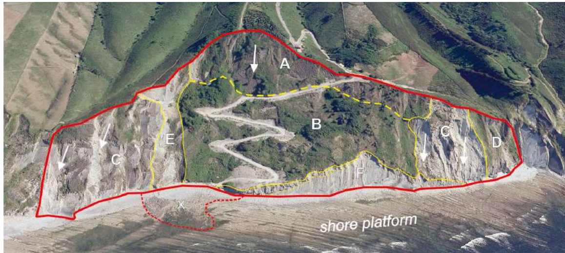
Figure 6 - Annotated Google Earth imagery (image dated 2011) of the complex Baratzarrak landslide showing its main units. Red line shows the extent of the entire landward part of the landslide area. A) head scarp; B) displaced blocks with stepped and hummocky topography; C) exposed slip planes of translational slides (sense of movement indicated by arrows) and minor perched patches of disintegrated bedrock; D) marginal part of the landslide, with slip planes largely overgrown; E) subsequent debris slides; F) landslide toe subject to marine undercutting and trimming. The dotted line separates landslide deposits (above) from intact bedrock (below). The area marked by 'X' within the shore platform shows considerable distortion and disintegration of flysch strata, interpreted as an effect of overload caused by landslide body, which extended father into the sea but was subsequently eroded.
