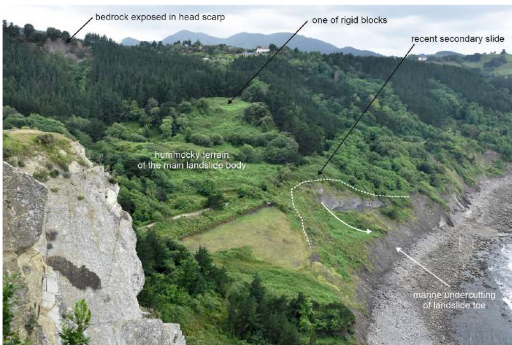
Figure 12 - Morphological details of the Mendatagaina landslide unit A (see fig. 11) which is extensively covered by vegetation. Secondary slides can be clearly seen in the toe part.
