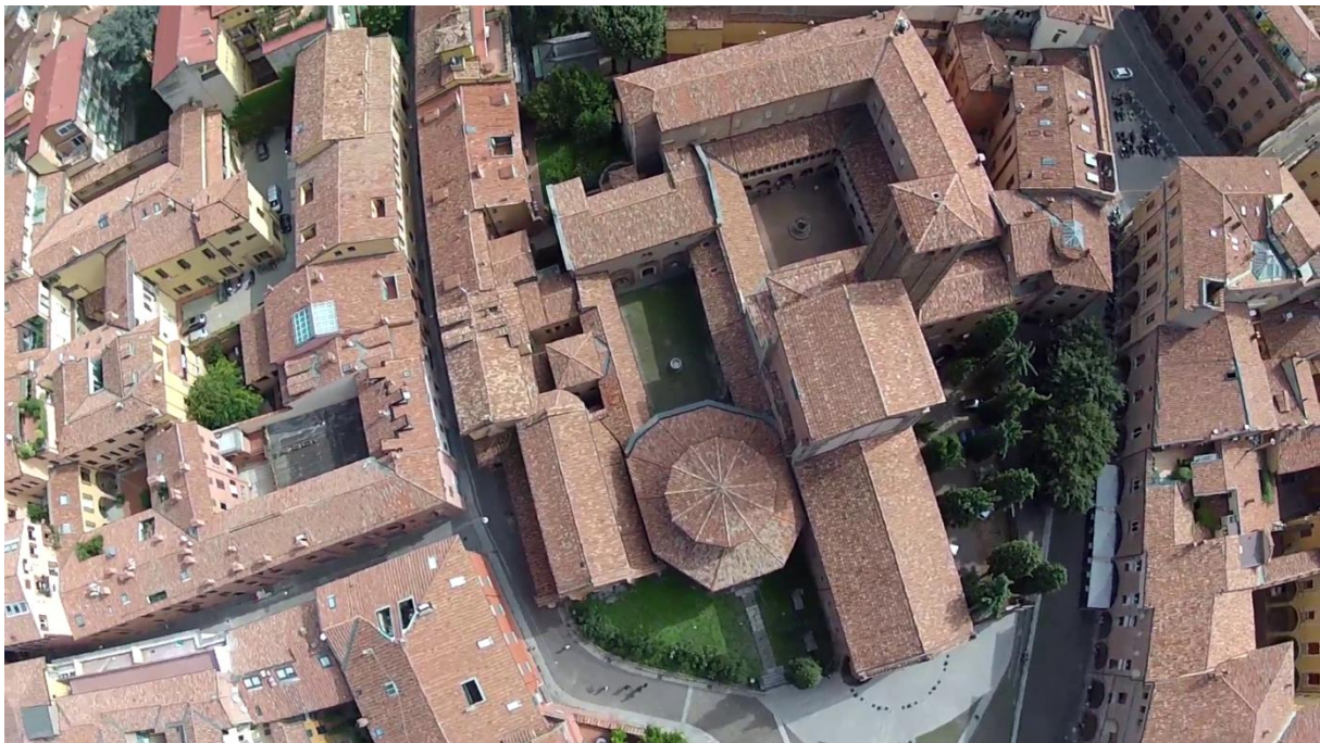
Figure 7.1 An overhead view of the Basilica Santo Stefano, Bologna (Italy)
