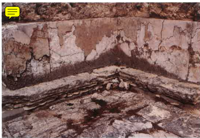
Fig. 1 – Partially dehydrated gypsum block (white, center) located in a wall structure at Eracle Minoa (Sicily). The other gypsum block immediately on the right is unaltered, whereas the thickness of the white surface decreases toward the right, suggesting that a fire burned the left side of the wall decreasing in intensity and effectiveness to the right. Note that the other adjacent rocks, arenite (deeply altered, at bottom) and limestone (left), do not show traces of burning. The gypsum blocks are about 30 cm high.
