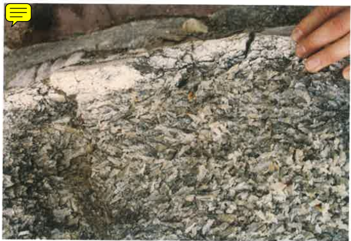
Fig. 4 – Close-up of the wall structure of fig. 3 (Palace of Minos, Knossos, Crete). Note that the white surface cut through blocks with different crystal orientations, indicating that dehydration occurred after emplacement of the blocks.
