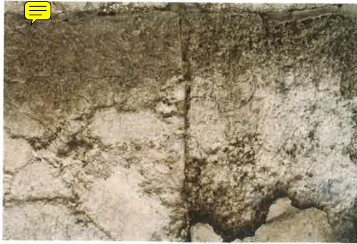
Fig. 3 – Partially dehydrated gypsum blocks (white) in the western façade of the Palace of Minos at Knossos (Crete). Note that the boundary of the white surface correlates across different blocks, indicating that the blocks were dehydrated after their emplacement. The lower portion of the gypsum blocks are unaltered (dark gray), suggesting that the socle may have acted as a sort of shield against the fire («shield shadow»). This interpretation is supported by the observation that the gypsum blocks are completely affected by the white surface in those tracts where socle is missing (not visible on picture). The gray areas on gypsum blocks are concrete restorations. Vertical blocks are about 60 cm high.
