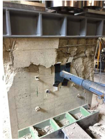
Fig. 20. Failure of the reinforced wall.
